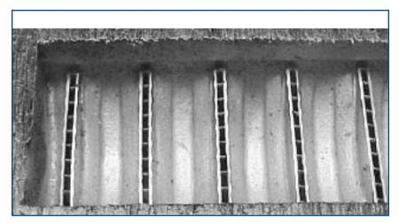
**Cutaway View of Parallel Flow Condenser Tubes**
