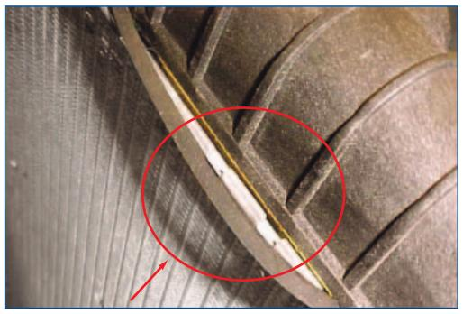
Blown gasket seam caused by excessive pressure
